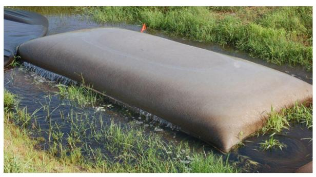
Figure 5.4 Example of Silt Dewatering Bag
