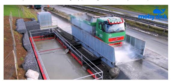
Figure 5.1 Example of Wheel Washing System
