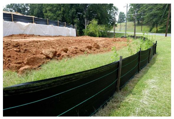
Figure 5.3 Example of Silt Fencing
